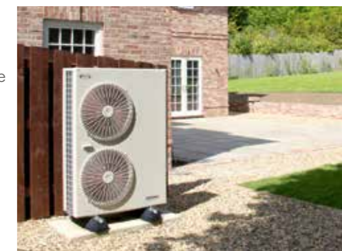
Above: Grant's Aeron3 13kW and 17kW air source heat pumps both hold Quiet Mark certification. Here, the external unit has been installed behind fencing for even greater acoustic protection
